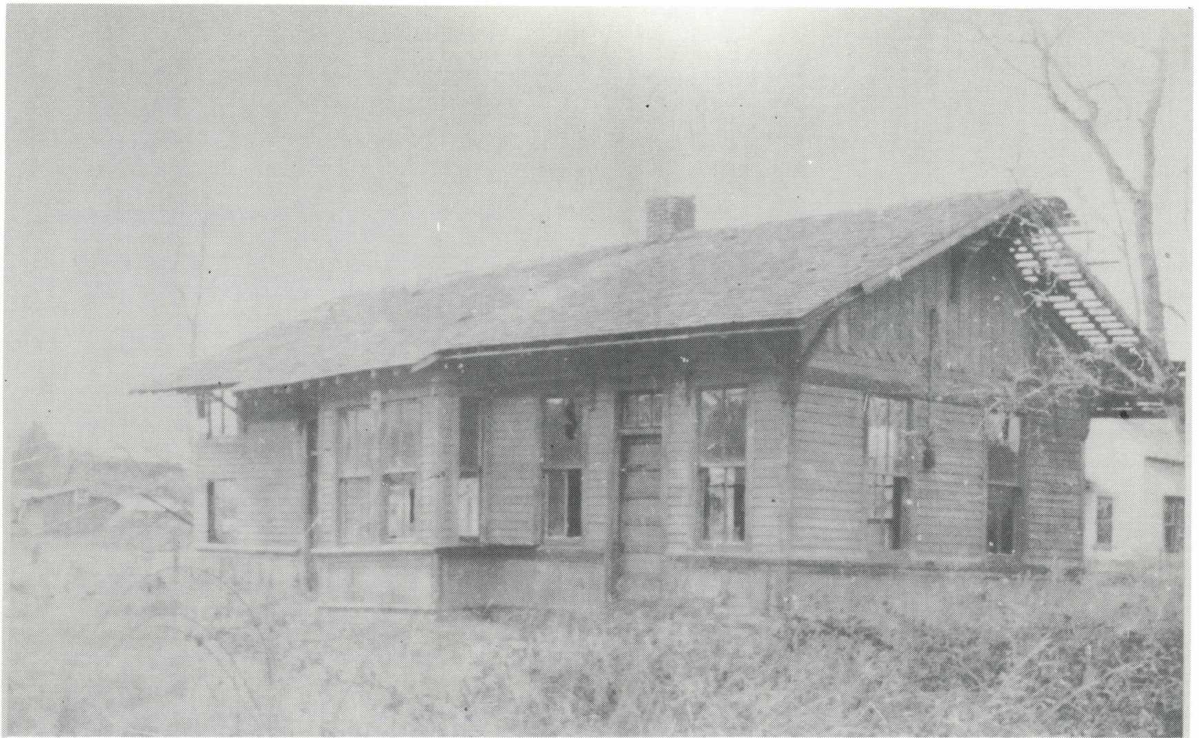
The Dryad depot was still in its orange and maroon colors, but sadly, looked every bit the relic it had become. Within two years of this photo, it was gone. - Alan Miller photo, April 12, 1975
